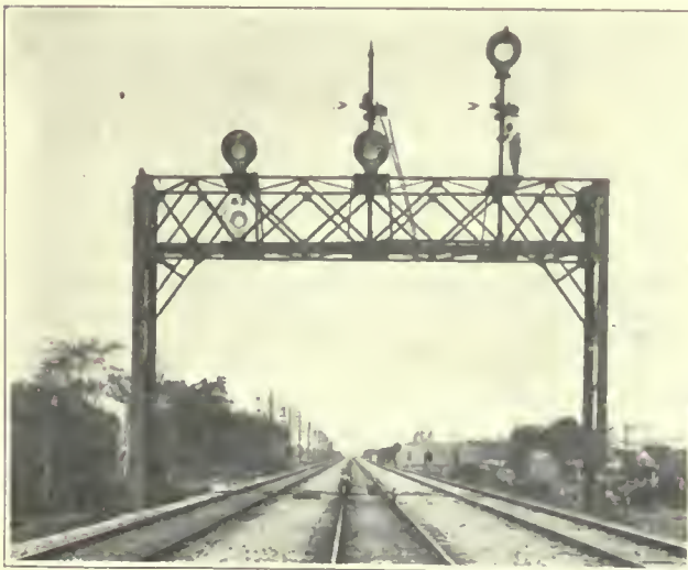
FIG. 286. SIGNALS. Signal bridge on the Chicago & North Western Railway, near Rosehill Station.
